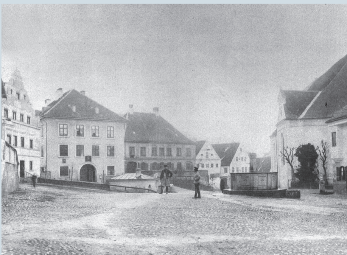
The County Magistrate's House (3rd left), around 1900
